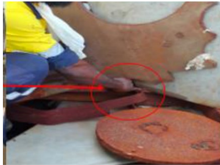
2: Dislodged Metal Plates
